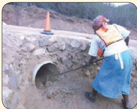
cleaning of pipe culverts
