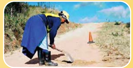
Zibambele contractor doing pothole patching along the road
