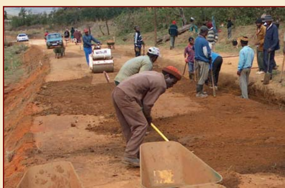
Labour intensive work in progress on the KwaGuqa Access Road
