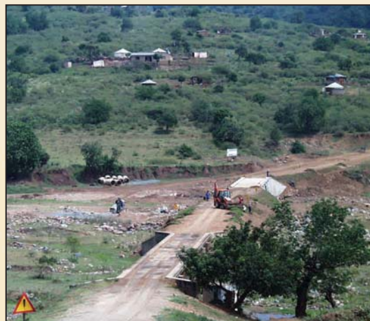
Almost complete new bridge in November 2002, tail end of earthworks remaining.
