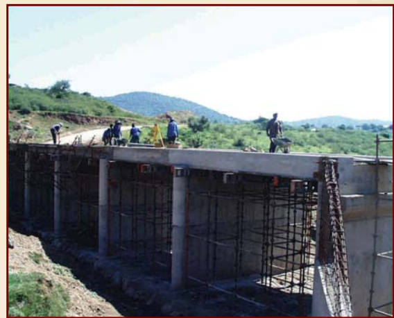
Mpisi River Bridge in October 2002.
