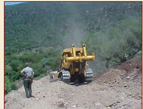
Nhlesi Road under construction in mountainous terrain
