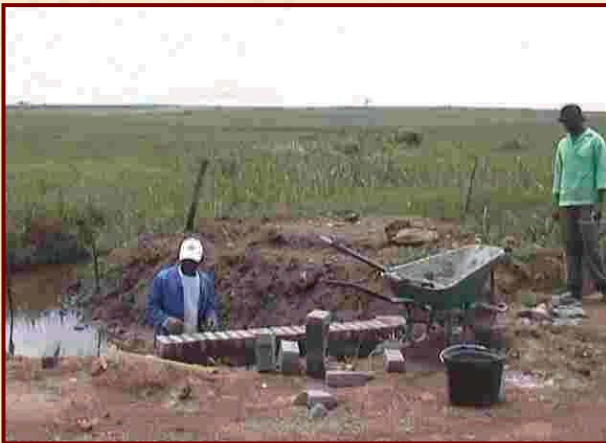
Belgrade Project: Headwall Construction
