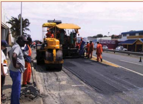
Roller and paver in action on site, after milling operation. October 2002
