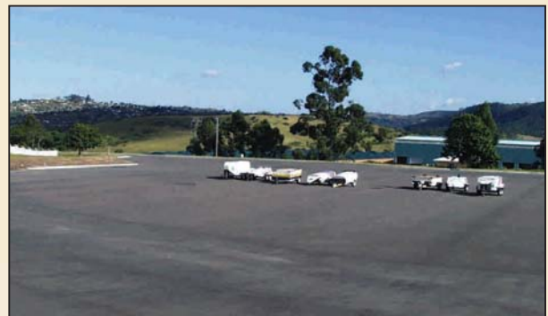
Vehicle impounding area strengthened to accommodate overloaded vehicles.
