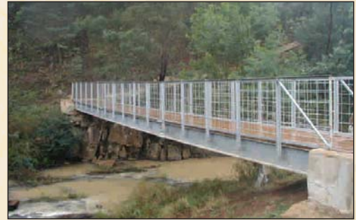
Foot Bridge over Umsunduzi River
