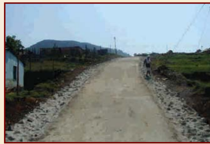
Stone pitching of side drains on the Fafaza Road
