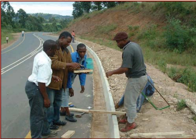
Do-It-Wise Construction receiving on-site mentorship on P100 ARRUP project
