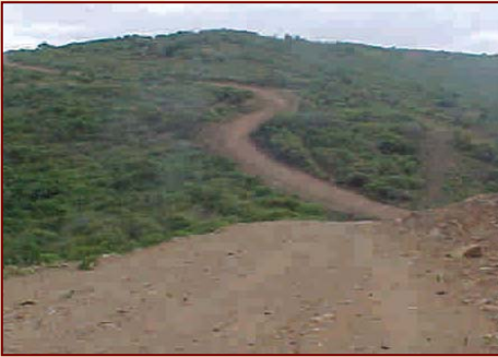
The new Mfithi Access road
