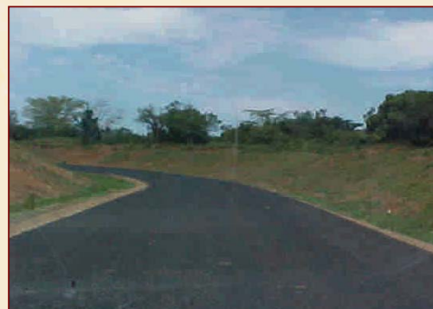
D 820 Linking Jozini to several towns on route to Mbazwana
