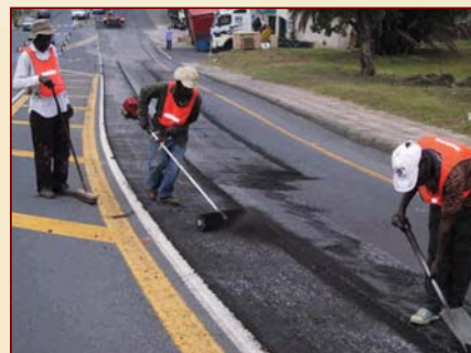
Road being swept after milling. October 2002
