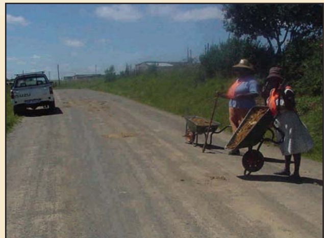
Zibambele Contractors : Pothole patching
