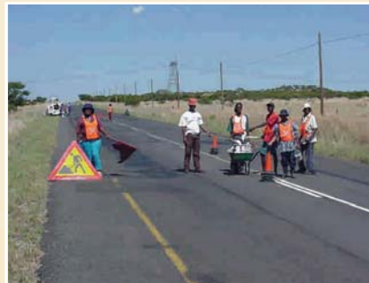
Initial Stage 1 Vukuzakhe Contractors carrying out manual road marking
