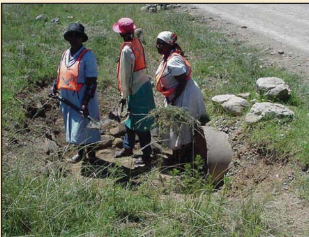
Zibambele Contractors: Drain Cleaning
