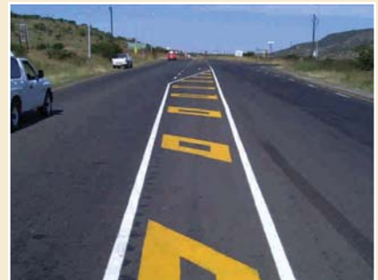
Completed road marking by emerging contractor in the Ladysmith Region
