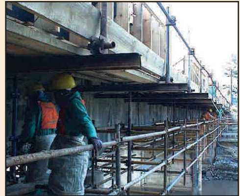
Workmen busy with construction on the underside of the deck
