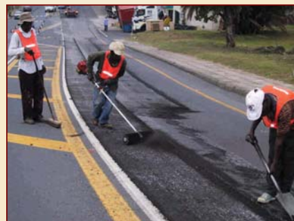
Road being swept after milling. October 2002
