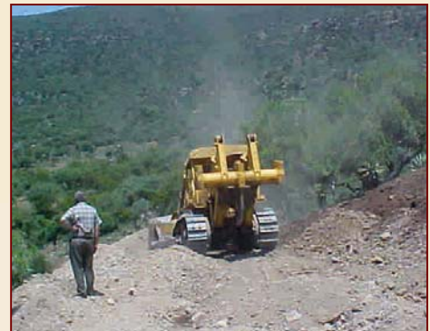
Nhlesi Road under construction in mountainous terrain
