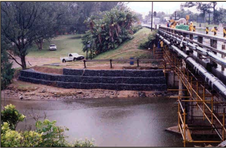
Side view of the Mzimayi River bridge on MR 3 Port Shepstone.
