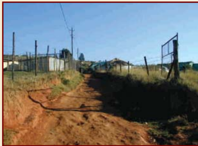
Fafaza Road prior to upgrading
