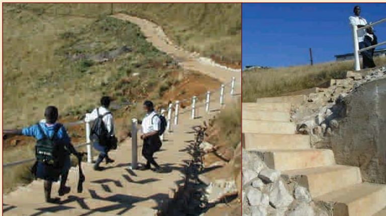
Mashingeni Staircase providing all weather access in the very steep terrain
