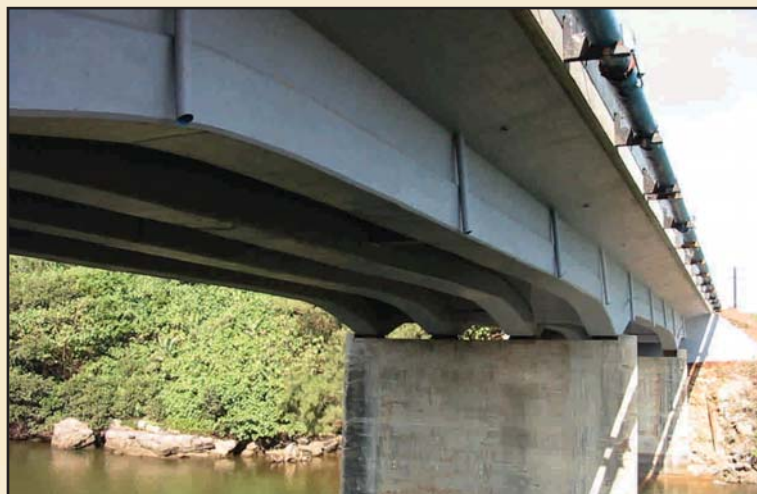
Underside of rehabilitated deck.
