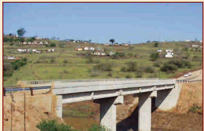
The new Umsunduzi River Bridge
