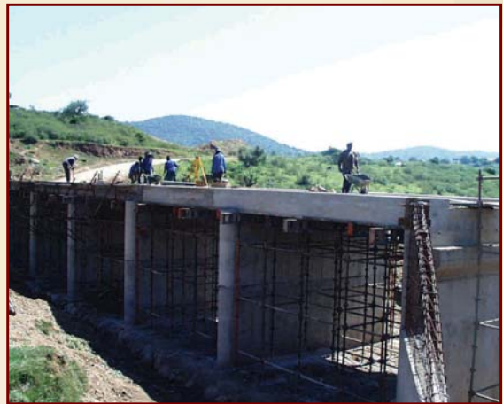
Mpisi River Bridge in October 2002.
