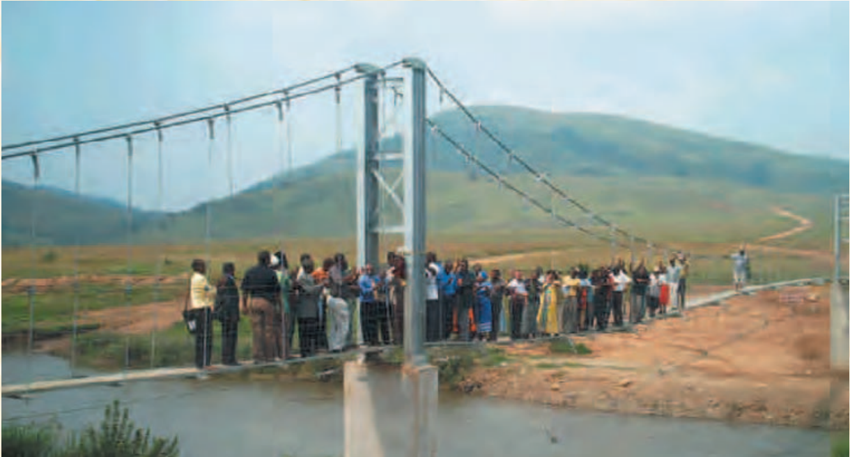
One of the Departments success stories: Obivane River Bridge.
