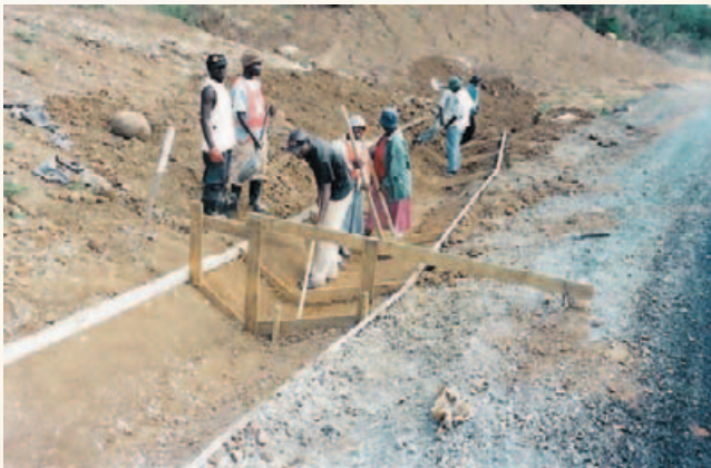
Technical training on the construction of Concrete V Drains on Main Road 235/2
