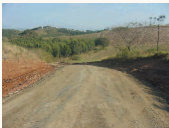
A completed section of the Iwangu road.
