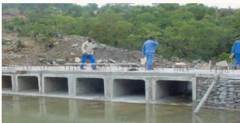
Structure on Mziyonke Local Road
