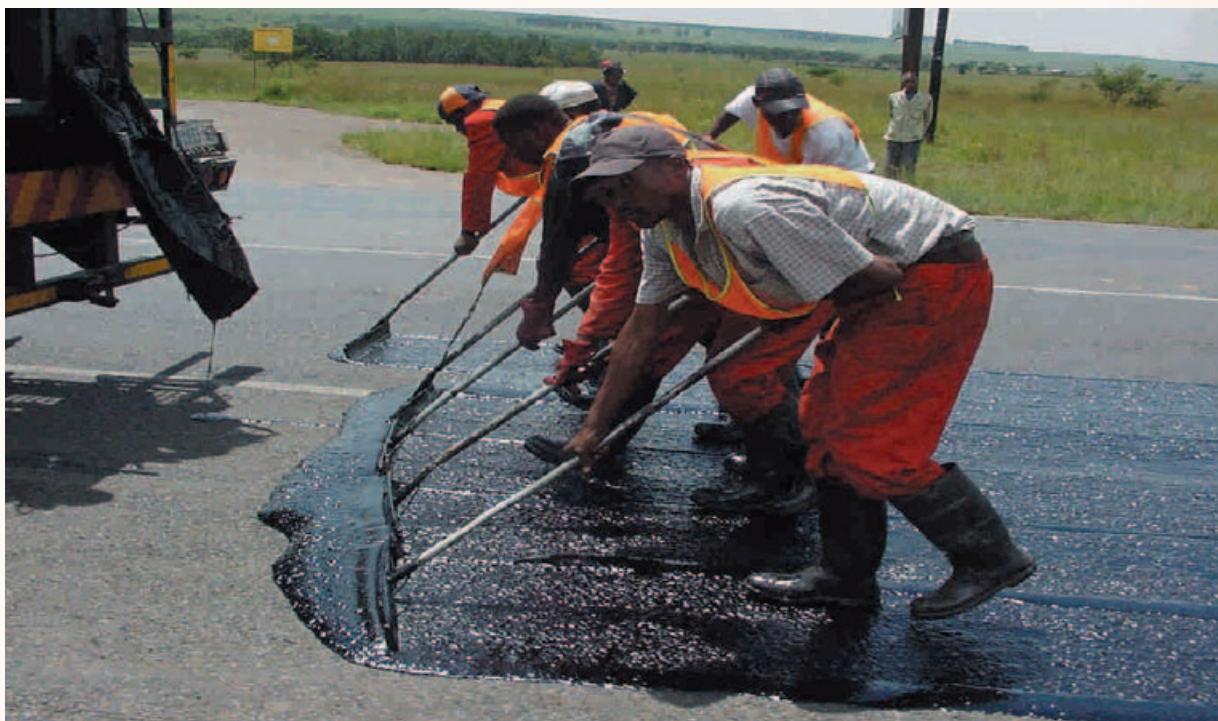
Team Spreading The SP2000 Rejuvenator On Main Road 10 – 1
