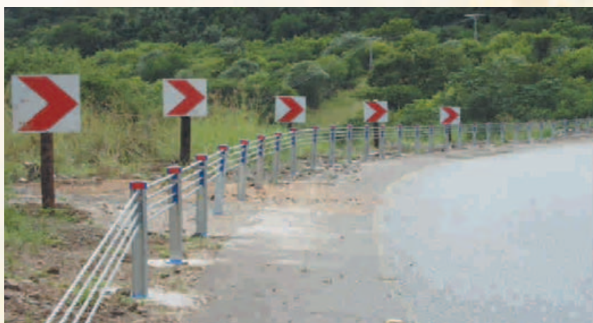
The new type cable guardrail between Ixopo and Umzimkhulu
