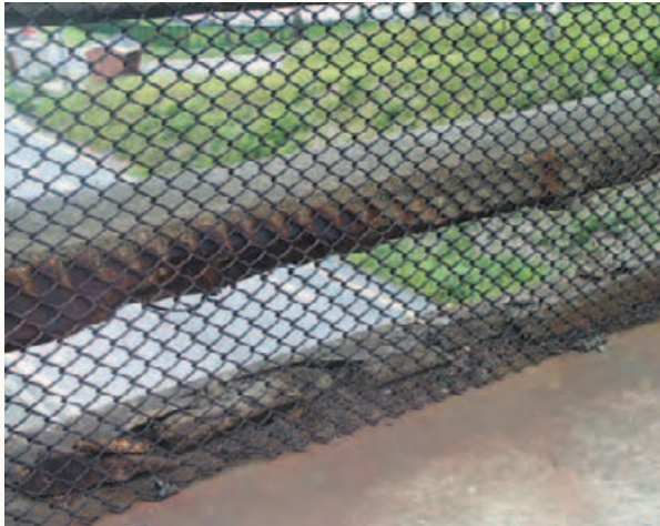
Prior to repair, showing corroded and cracked concrete elements
