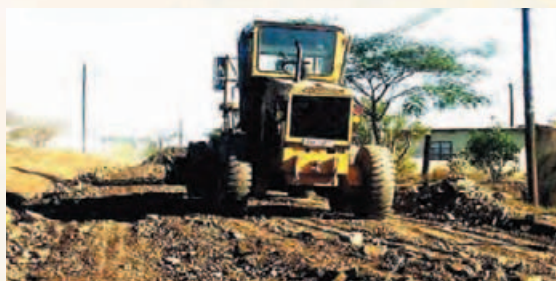
A Departmental grader spreading gravel on the Khovoti Road prior to gridding
