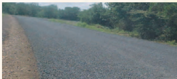
A newly surfaced section of D820
