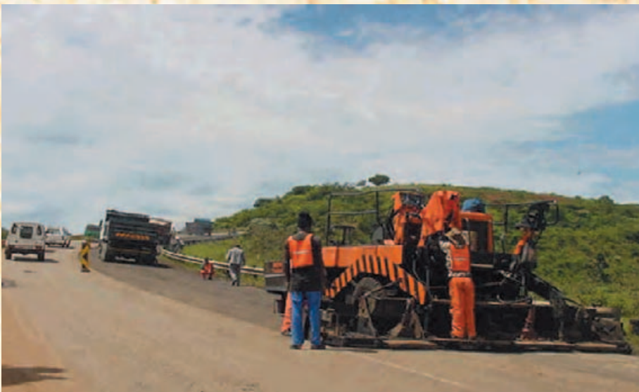
Paving of the asphalt layers
