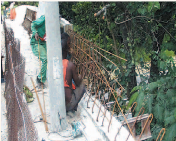
The New Jersey Parapets During Construction
