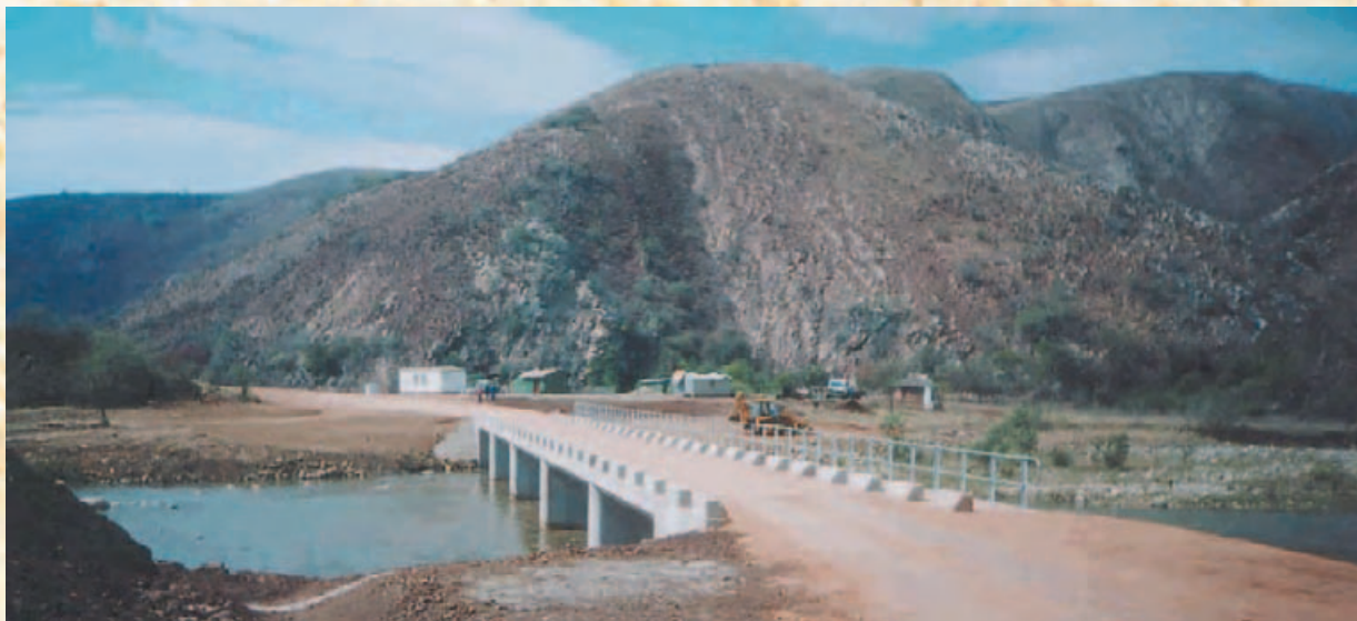
The completed bridge over the Nsuze River on Main Road 90
