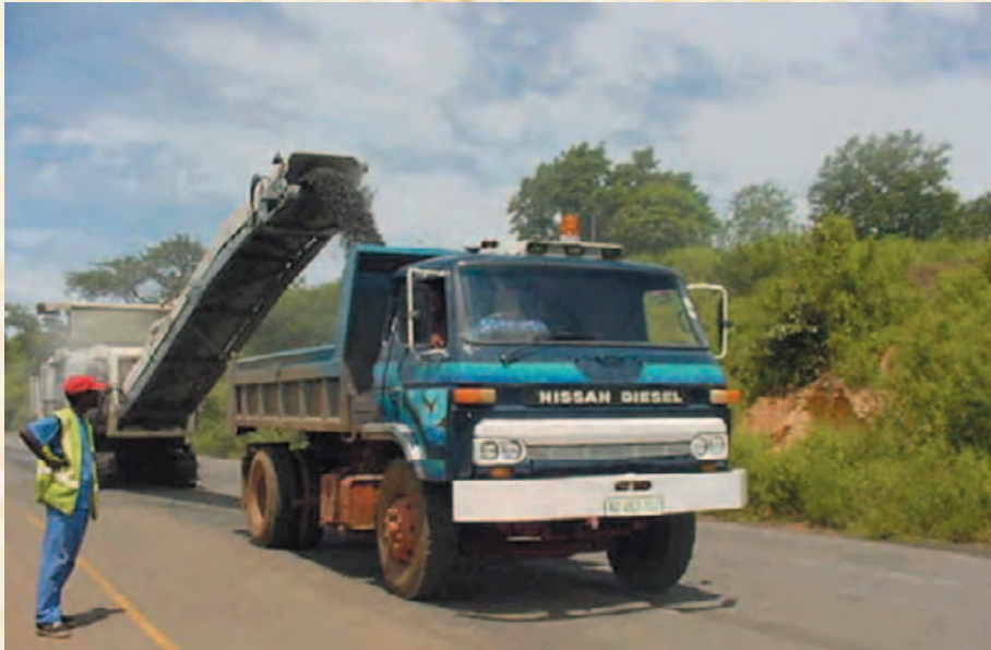
Milling work in progress
