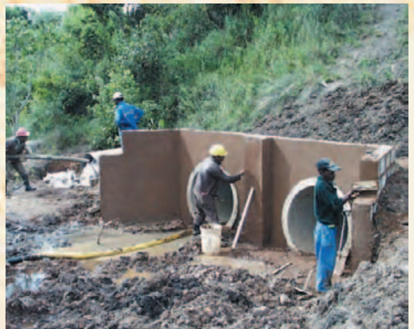
Grouting and Construction of Headwalls
