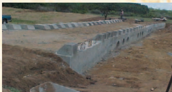
The Ezinsileni Causeway nearing completion on the Ubumbano Road
