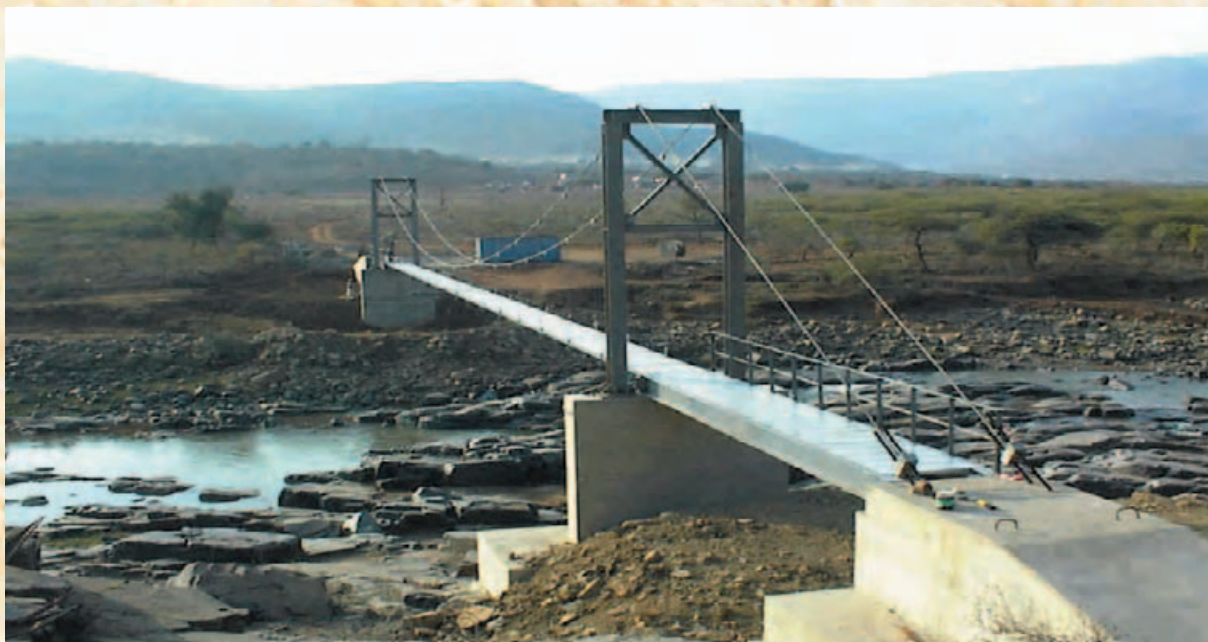
Pedestrian bridge over the Mooi River
