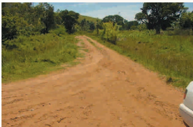
The Iwangu road before upgrading
