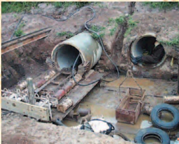
P21-2: Pipe jacking in progress
