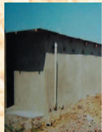
New Toilet Block
