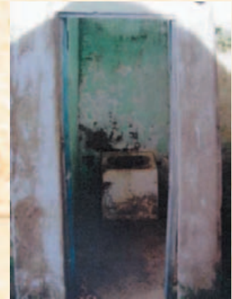
Old Toilet Block
