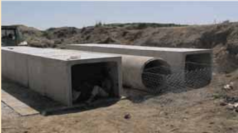
Pitout Causeway DC25 in Utrecht during Construction
