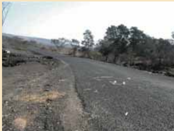
Road D173 Before Resealing
