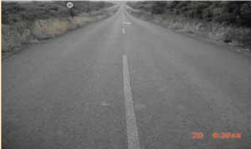
Portion of upgraded P 236
