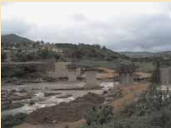
D1000 Bridge: During Construction
