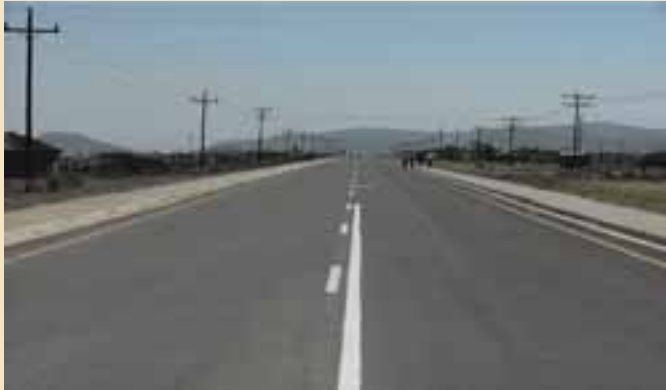
Completed section of Road P700
