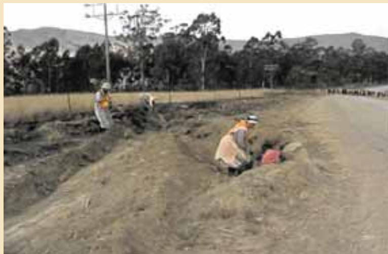
Zimbabwe Road Workers Opening Up Drains
