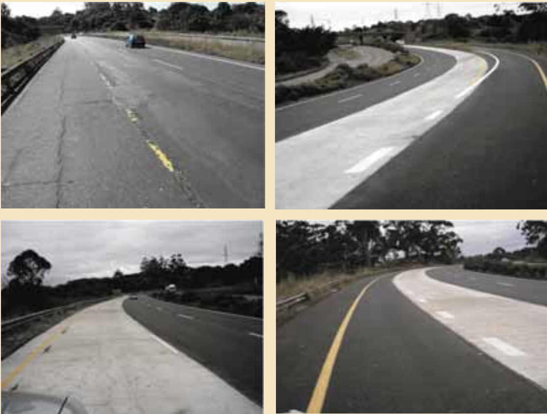
Sections of Road P82 During Rehabilitation
