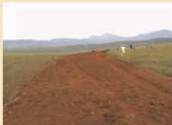
Completed portion of Thwabala Road
