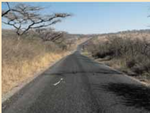
Road D173 After Resealing
