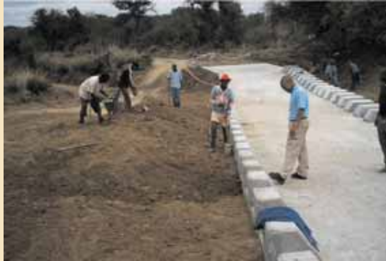
Siphandule Causeway in Pongola during construction
