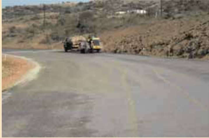
Umsimbiti Base Course Construction on site
