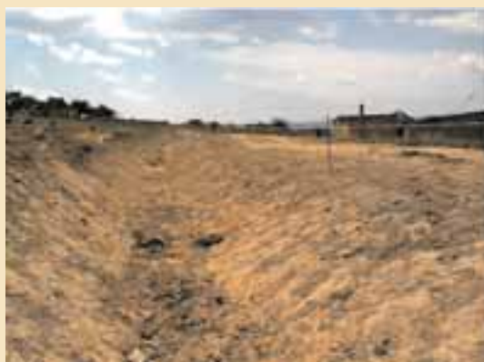
Thwabala Road during construction
