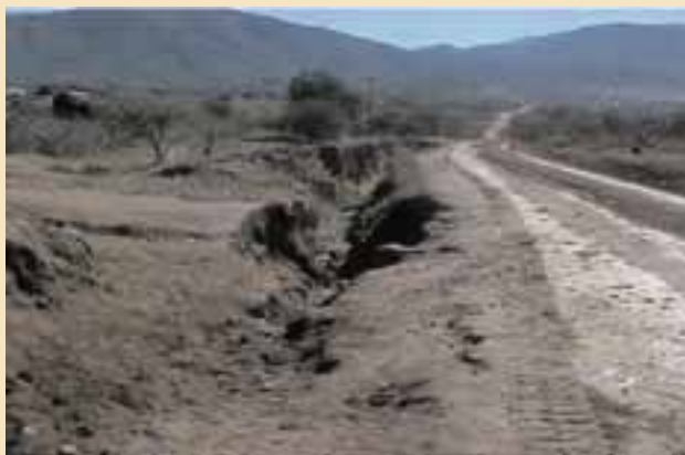
Road D1639 before reshaping of the road
