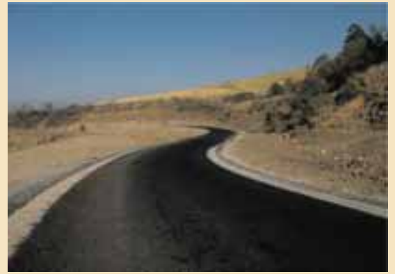
Road P26: After Construction
