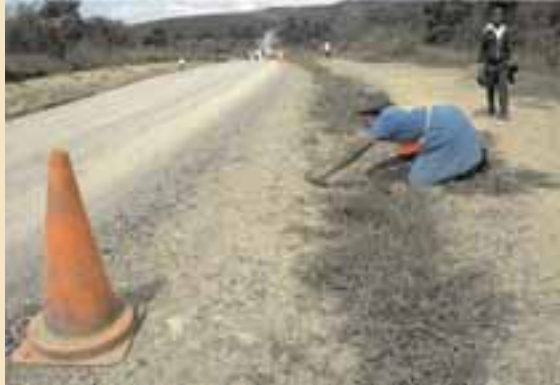
Zimbabwe contractors clearing drains along D1133 known as (KwaNzokane Loop Road) in the Vulindlela RRTF area, Pietermaritzburg
