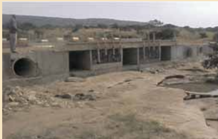
Doornkop Causeway During Construction
