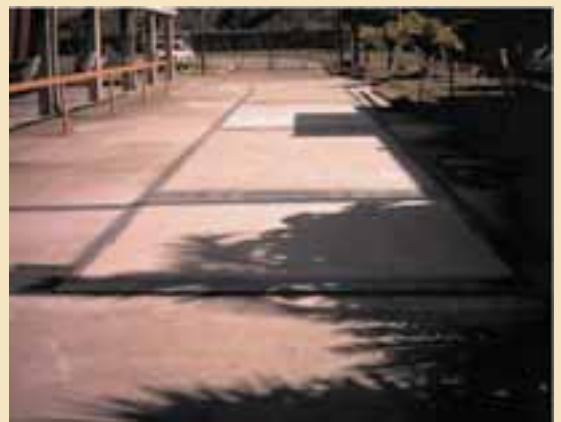
After: Marburg Concrete Multi-deck
