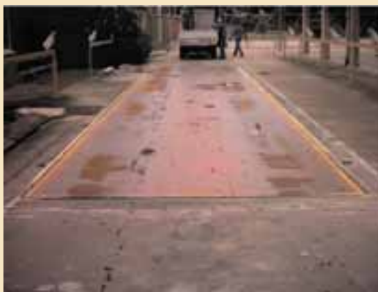
Before: Marburg Weighbridge
