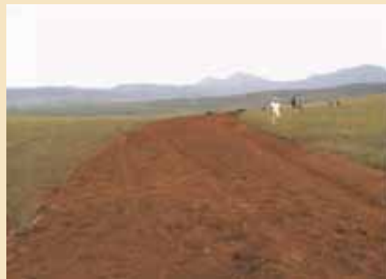
Completed portion of Thwabala Road
