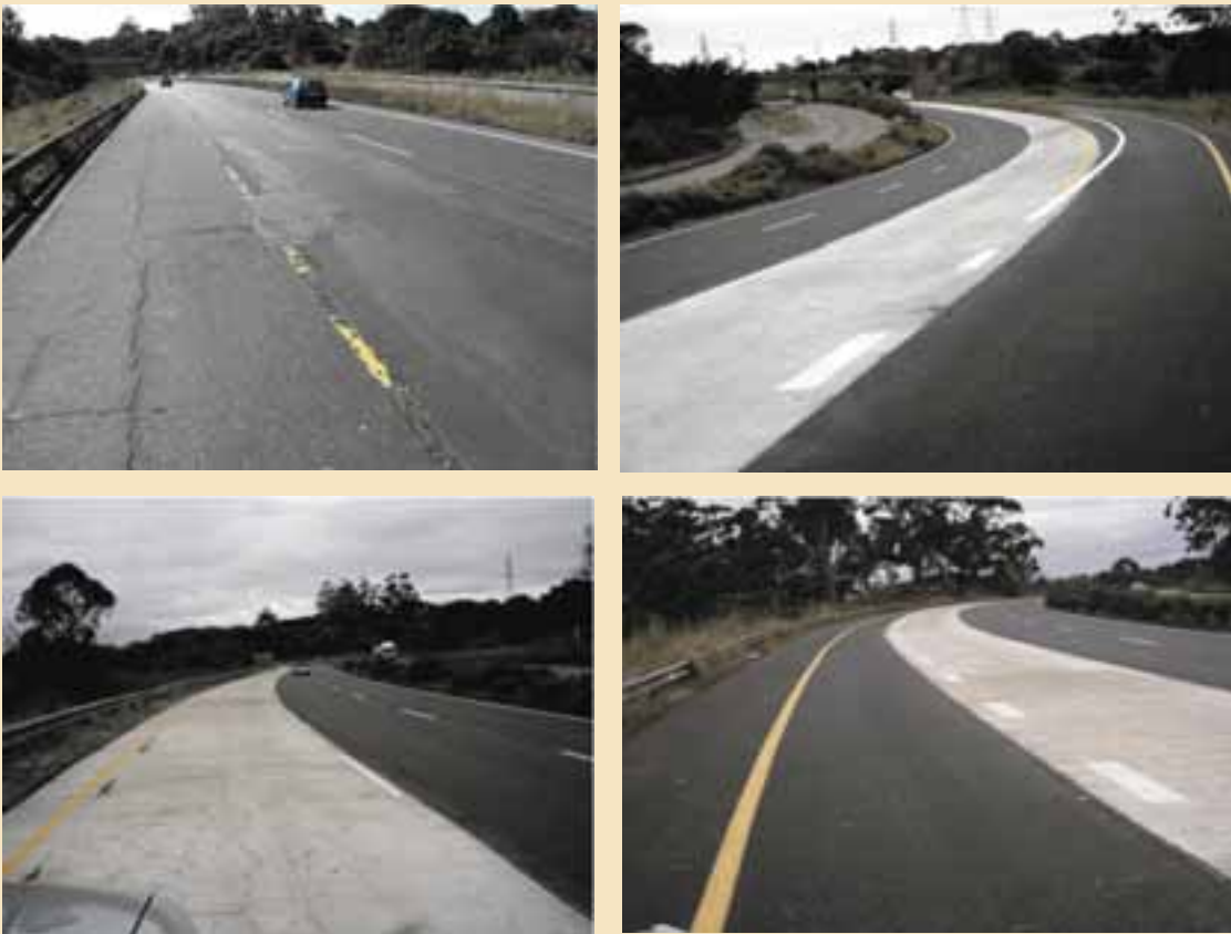
Sections of Road P82 During Rehabilitation
