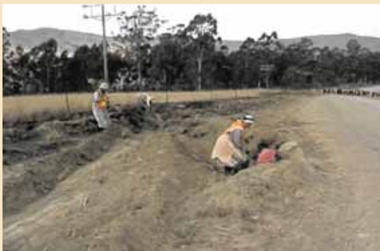
Zimbabwe Road Workers Opening Up Drains
