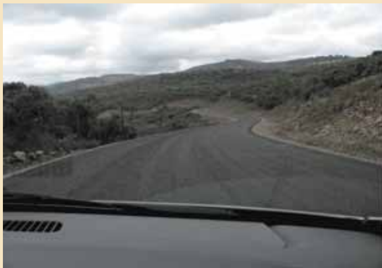
Road D1820: After Construction
