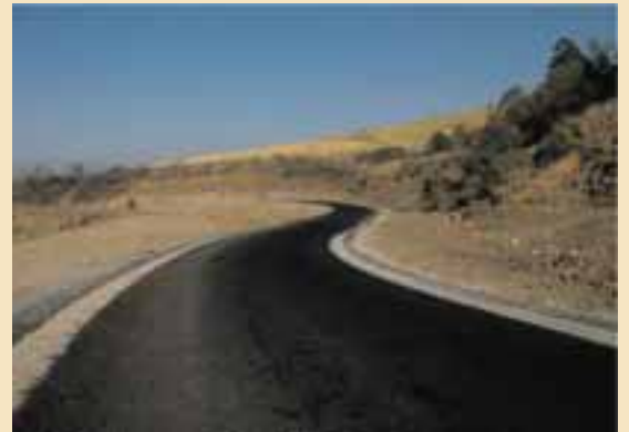
Road P26: After Construction
