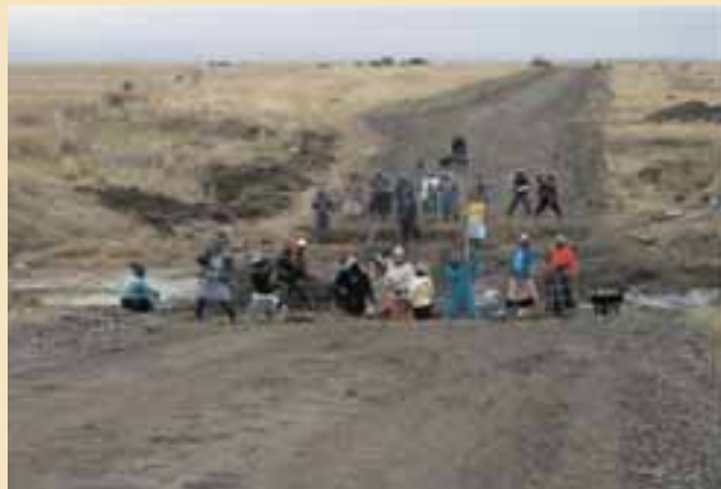
Community workers digging a trench for causeway at Mnxangala Road (Nquthu RRTF)
