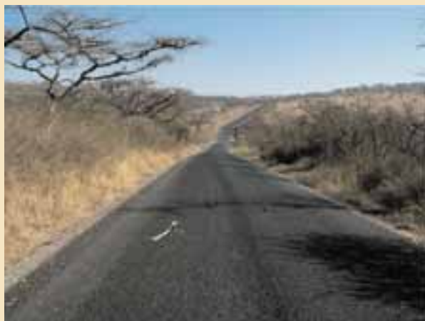
Road D173 After Resealing
