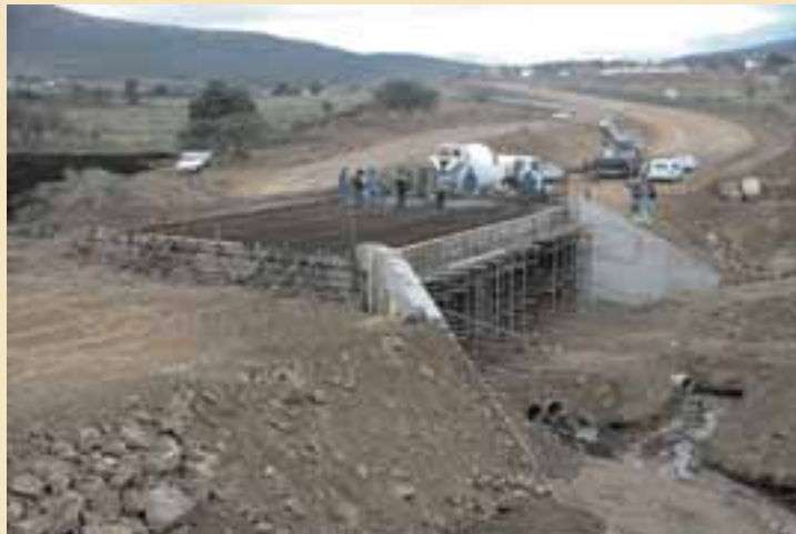
Mpuze River Bridge Under Construction
