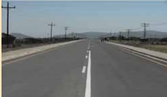
Completed section of Road P700
