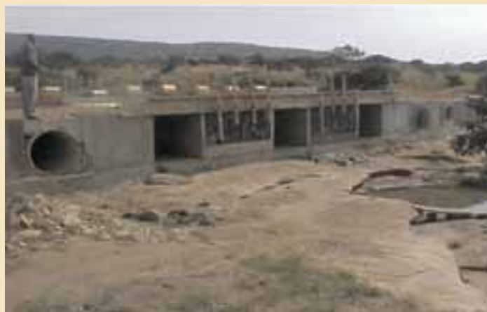
Doornkop Causeway During Construction
