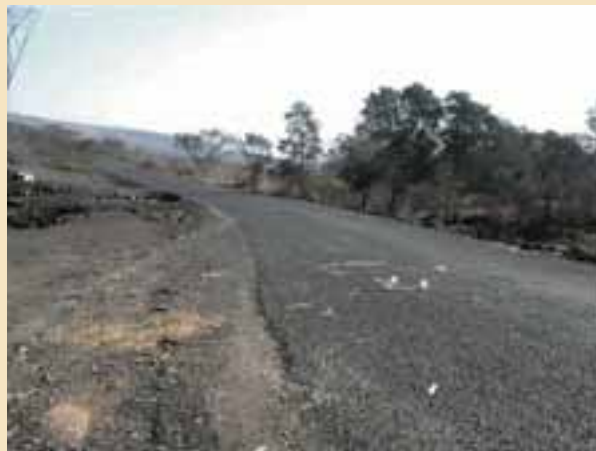
Road D173 Before Resealing
