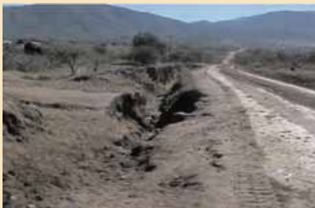
Road D1639 before reshaping of the road
