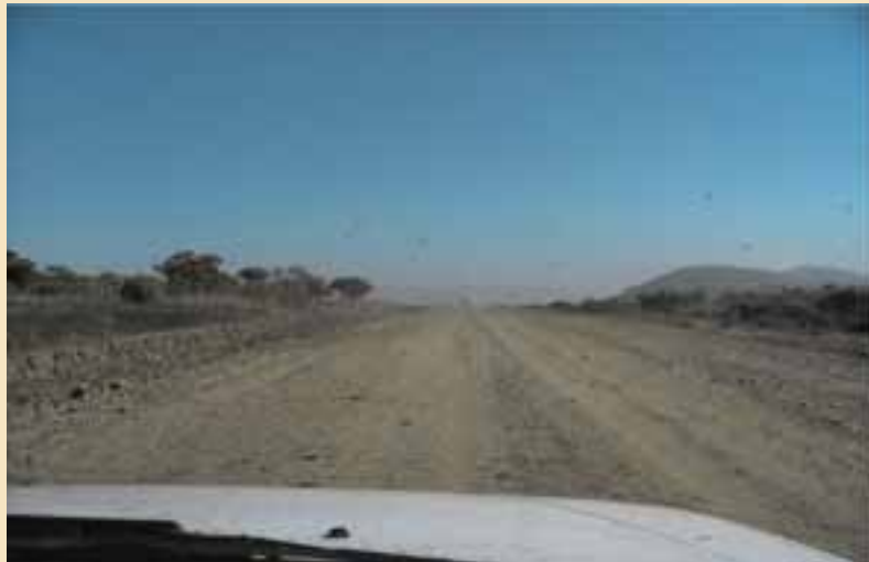
Road D1820: Before Construction
