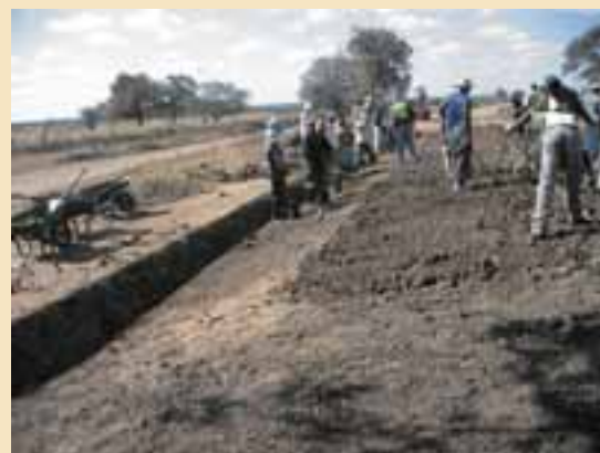
Community workers opening up side drains at Mkonjeni Road (Jozini RRTF)
