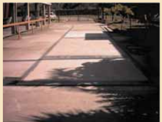
After: Marburg Concrete Multi-deck
