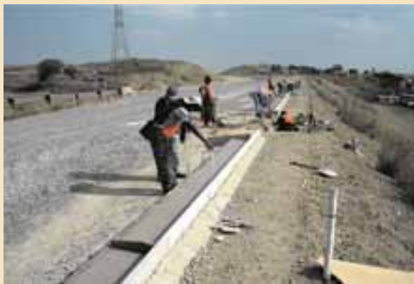
Construction of kerb and channel on P577
