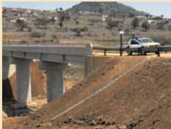
D1000 Bridge: Complete
