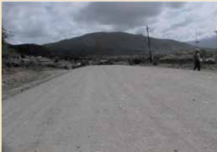
Road D1639 after reshaping of the road
