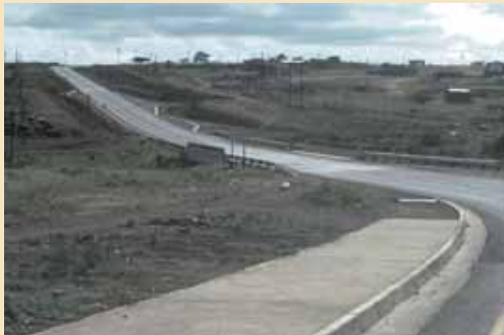
Road P700 Nearing Final Completion
