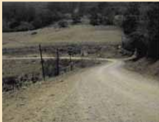
Road P26: Before Construction
