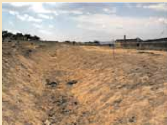
Thwabala Road during construction
