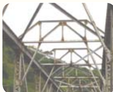
Rusted bearers and support & corroded parts of the bridge
