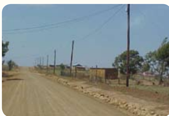
Portion of road D69 after regravelling
