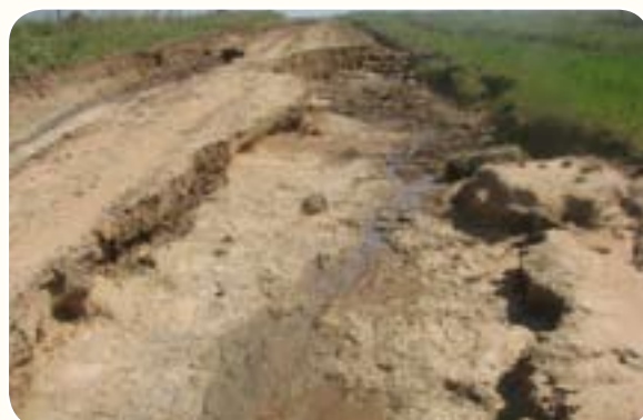
Erosion on road D332
