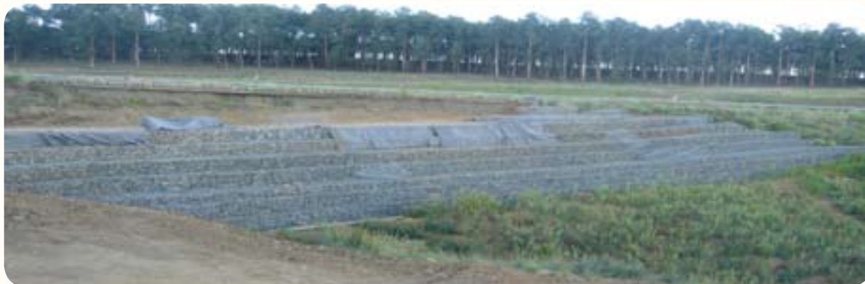
The gabion construction on P211 embankment
