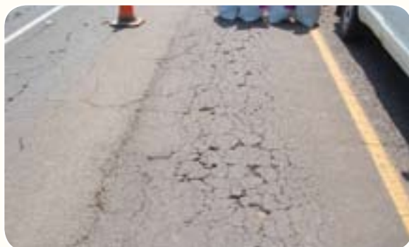
Cracks on portion of road MR34/3
