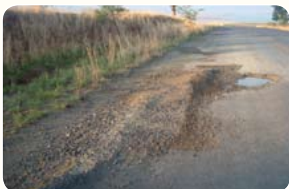
Portions of pothole patching, filling of material and compacting in progress
