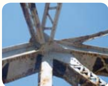
Rusted bearers and support & corroded parts of the bridge
