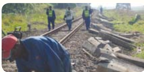
Labour-intensive rehabilitation of the Nkwalini line
