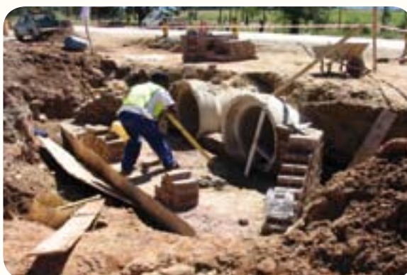
Pipeheadwalls settings & earthworks in Sani Pass Road during construction
