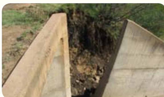
Collapsed wing walls of road P42
