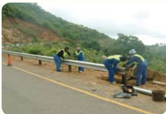
Some of the CETA learners, NQF level 2; installing guardrails
