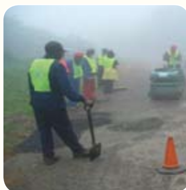
Pothole patching in progress
