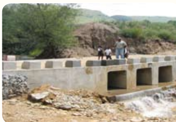
Funwayo causeway during and after construction
