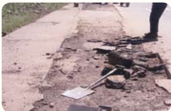
Pothole patching in progress
