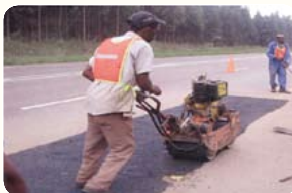
Pothole patching in progress
