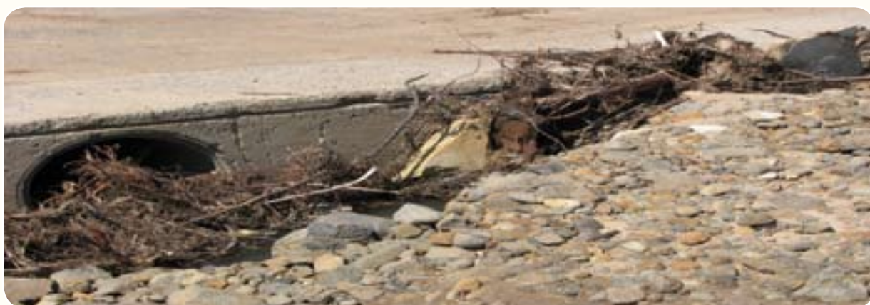
Blocked causeway on road D93
