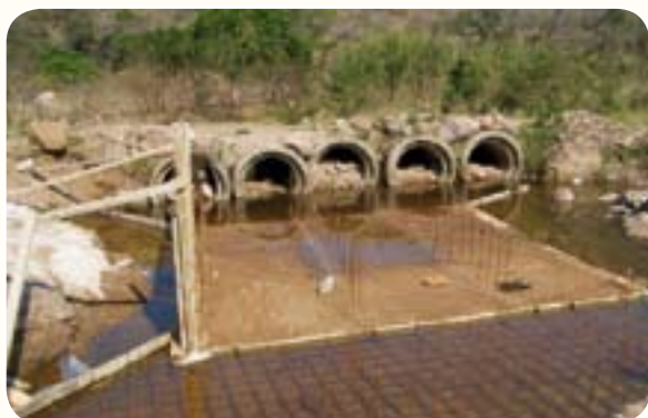
Molweni 2 causeway during construction
