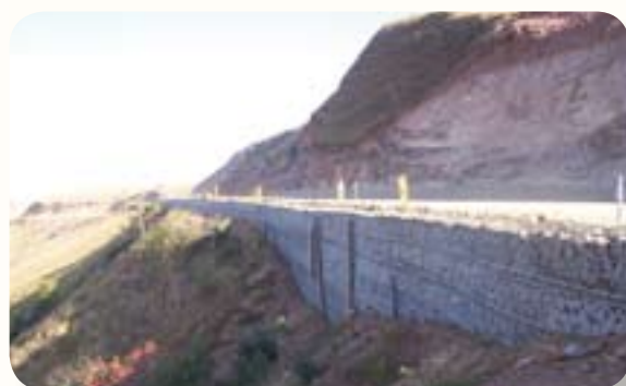
Retaining wall in difficult terrain on the P50/2 Inkandla Project
