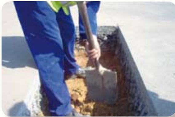
Installation of a Weigh-in-Motion (WIM)
