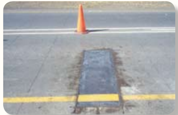
Installation of a Weigh-in-Motion (WIM)
