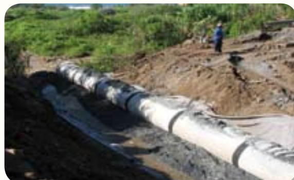
New pipe being installed
