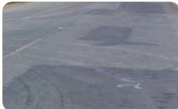
Before and after patching -P160
