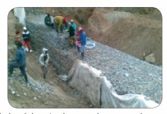
Construction of Gabion baskets at D634 where banks had eroded causing damage to the access roads
