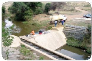
P235-2 Weir, complete with environmental fish ladder, constructed for the road-works and used by the local people
