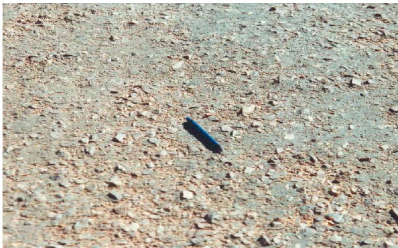
Figure 5: Appearance of a crushed rock section one week after construction.
