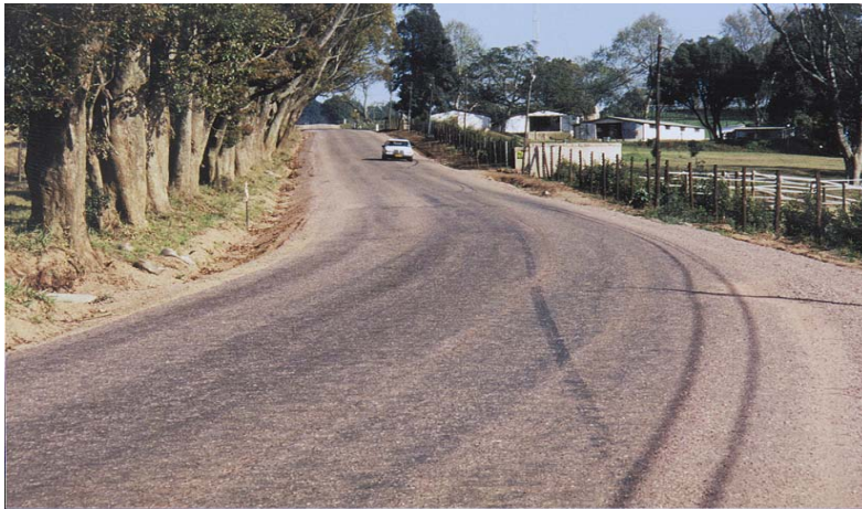
Figure 6: Characteristic premix look of Otta seal two months after construction.
