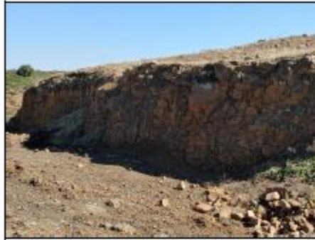
Figure 4. General view towards the west at existing cut
