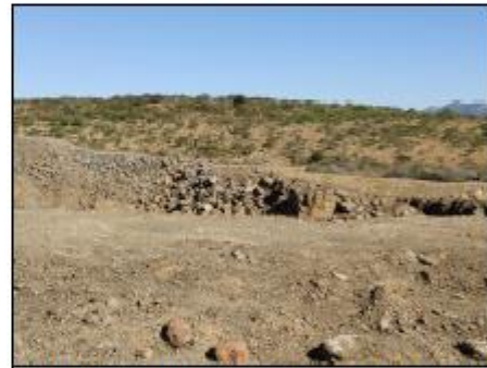
Figure 7. General view of borrow pit floor and previous subsurface excavations
